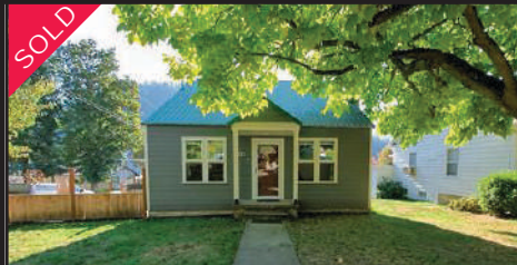
Beautiful home with many updates. New siding and most windows, some plumbing and electrical. Updated kitchen. Located within walking distance to downtown Orofino! 3 bd, 2 ba! $239,000 98862490
